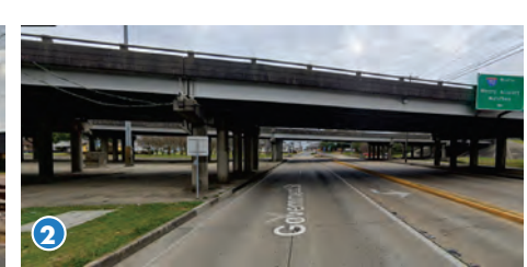
I-110 Underpass at Government Street
