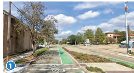
East Boulevard 1 Lane, Major Collector [low traffic, bike trail and sidewalks on either side, walkable]
