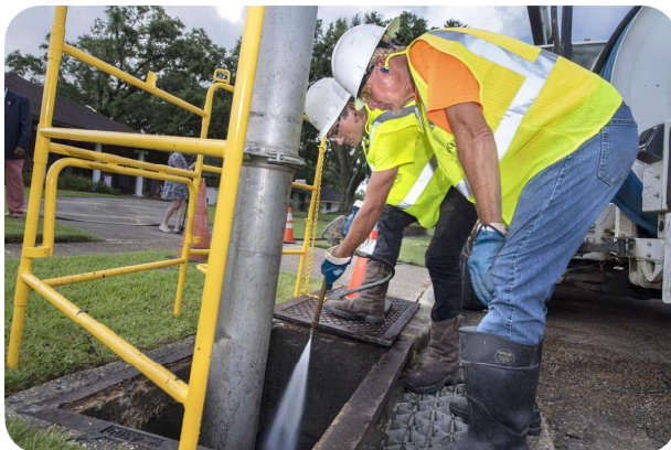
City-Parish workers clean a storm drain on Jefferson Highway
