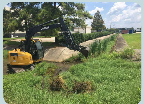
City-Parish workers clear a section of a canal Source: WAFB
