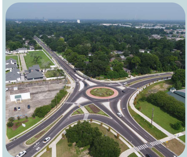
Before and after aerial photos of Government Street at Lobdell.
