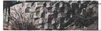
PROPOSED SPLIT FACED CONCRETE MODULAR RETAINING WALL WITH VARYING HEIGHT (MAX 5')
